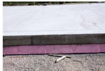
Figure 4: Floor slab with insulation layer (source: Schulze Darup)
