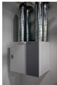
Figure 7: Convenience ventilation system with heat recovery (source: Bin im Garten;
