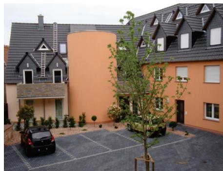
Figure 11: Solar house compound with solar storage unit (source: Andol; [http://commons.wikimedia.org/wiki/File:Solarhauskomplex\\_mit\\_Solartank.png#/media/File:Solarhauskomplex\\_mit\\_Solartank.png](http://commons.wikimedia.org/wiki/File:Solarhauskomplex_mit_Solartank.png#/media/File:Solarhauskomplex_mit_Solartank.png))
