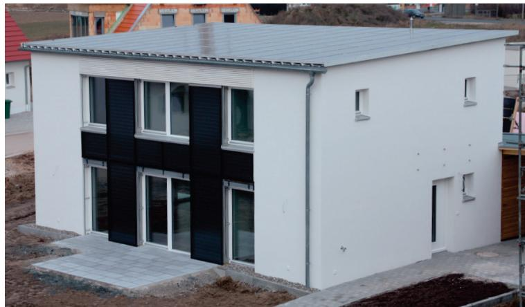
Figure 2: Example of a “Nearly Zero-Energy” building with photovoltaic system on roof and solar thermal system on front façade (source: Arch Wimmer – schulze darup & partner)
