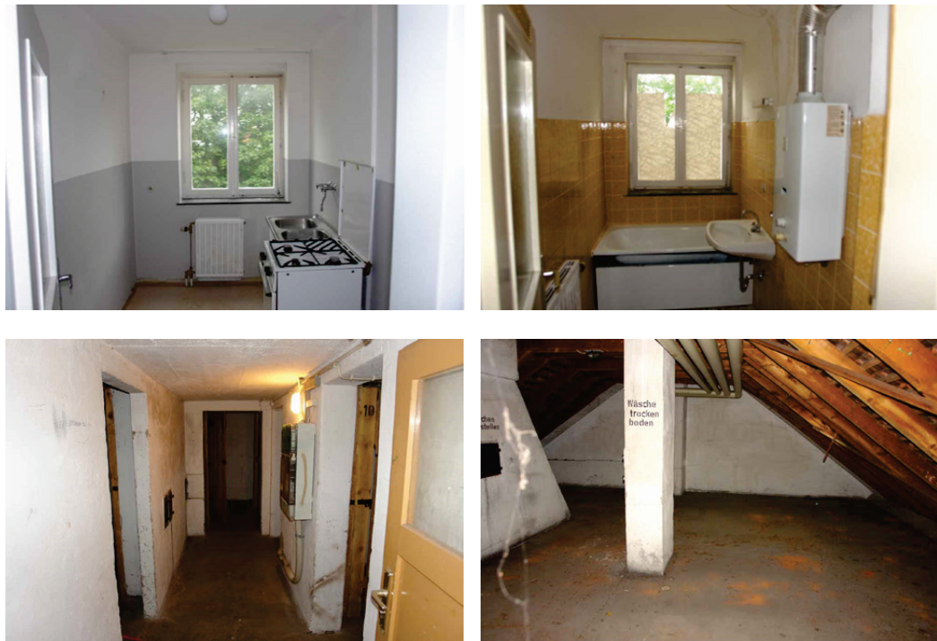
Figure 2: Apartment building before thermal renovation (source: Schulze Darup)
