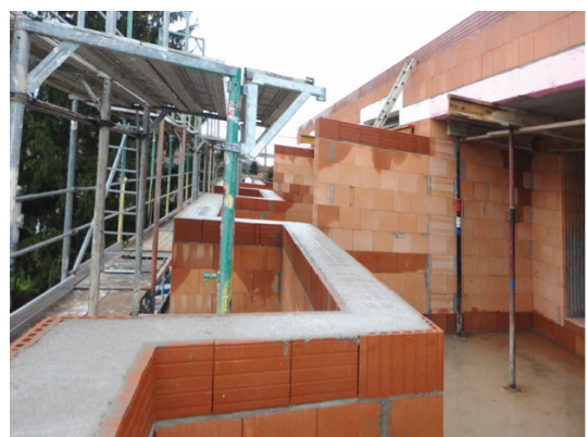
Figure 10: Single-shell brick masonry for a passive house (source: Schulze Darup)
