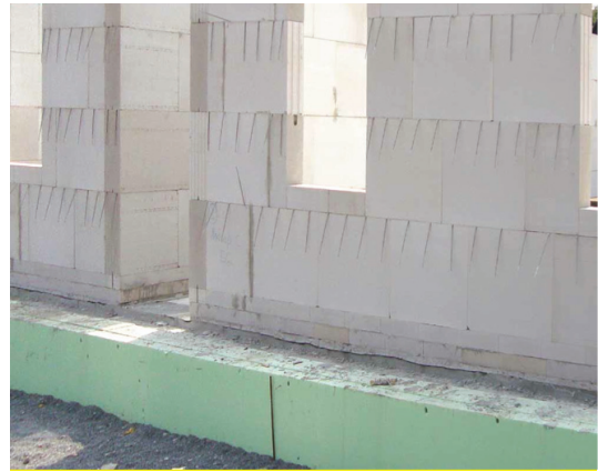
Figure 11: Inner masonry shell with wall anchors for the façade shell (source: Schulze Darup)
