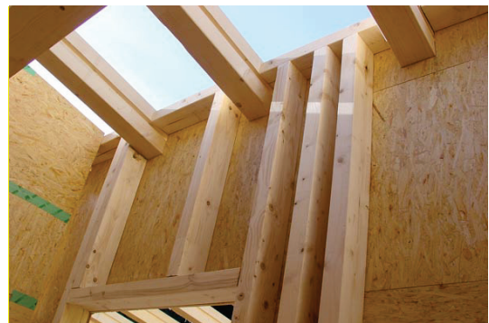
Figure 6: Timber frame structure (source: Holka Genossenschaft)
