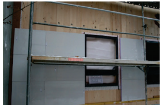
Figure 7: Vacuum insulation on a non-frame timber wall; cladding is provided by a curtain wall (source: Variotec, Neumarkt)
