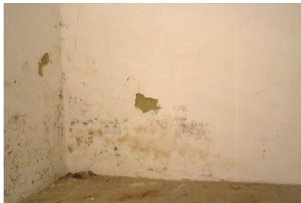
Figure 17: Mould developing in corners that form thermal bridges (source: GrAT)
