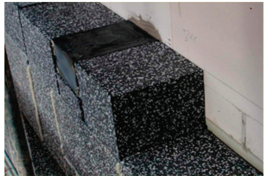
Figure 8: ETICS insulation with an anchoring point (implemented to minimize thermal bridging) for a light (source: Schulze Darup)
